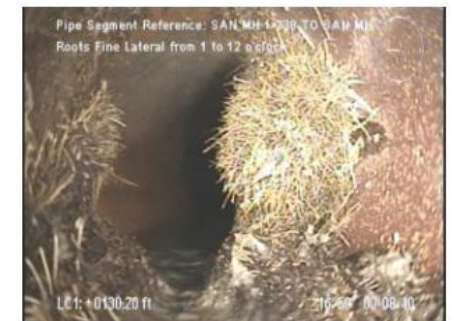
MH 1-238 to MH 1-237 Roots through joints
