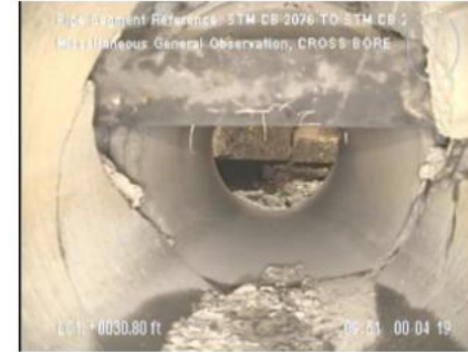
CB 2076 to CB 2075 Cross bore holes, fractures
