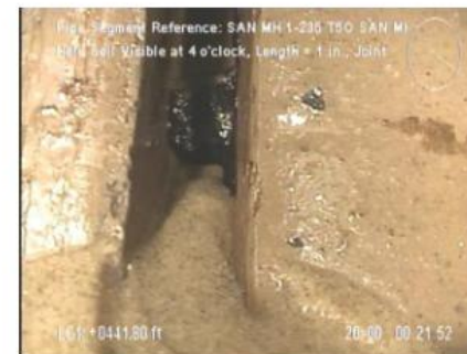
MH 1-235 to MH 1-234 Holes soil visible
