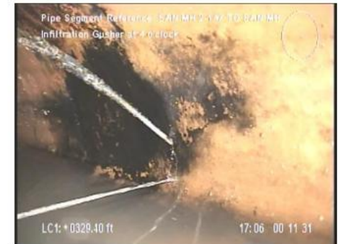
MH 2-147 to MH 2-146 Infiltration, cracks
