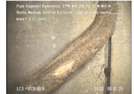
MH 255 to MH 45 Roots through joints
