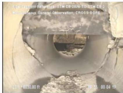
CB 2076 to CB 2075 Cross bore holes, fractures
