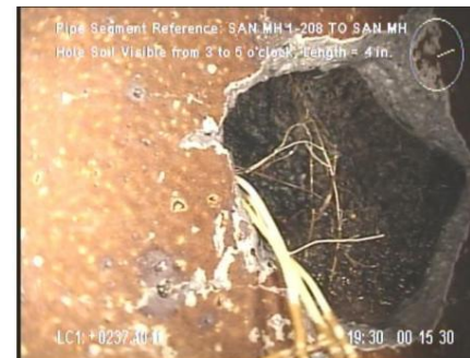
MH 1-208 to MH 1-210 Holes and roots, soil visible
