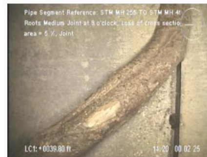
MH 255 to MH 45 Roots through joints
