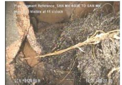
MH 4-036 to MH 4-055 Soil intrusion, roots and cracking
