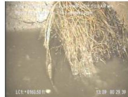
MH 3-011 to MH 4-036 Roots, cracks at joints
