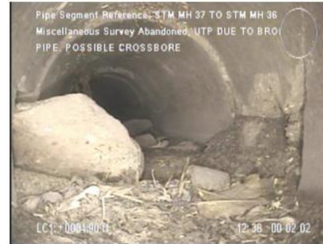
MH 37 to MH 36 Broken pipe, soil intrusion, holes
